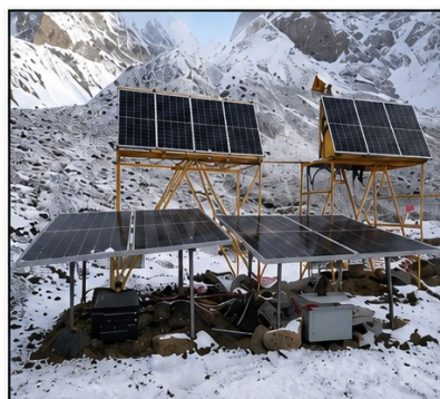
(b) Solar array powering continuous power supply to field instrumentation
